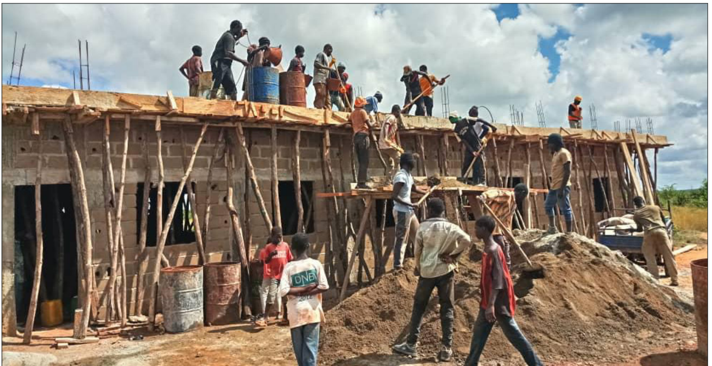
Holy Quran Hafiz School for Children Construction Site
