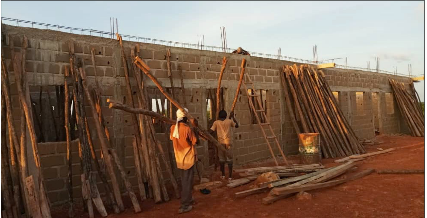
Construction of the Holy Quran School
