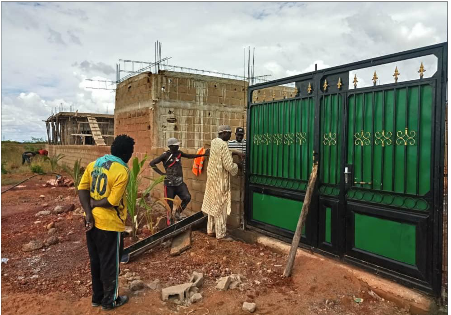
Holy Quran Hafiz School Construction Site in Bamako, Mali
